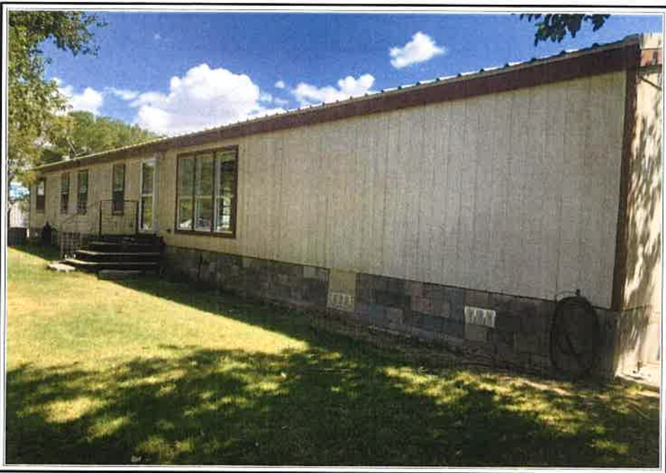
REAR OF SUBJECT PROPERTY
