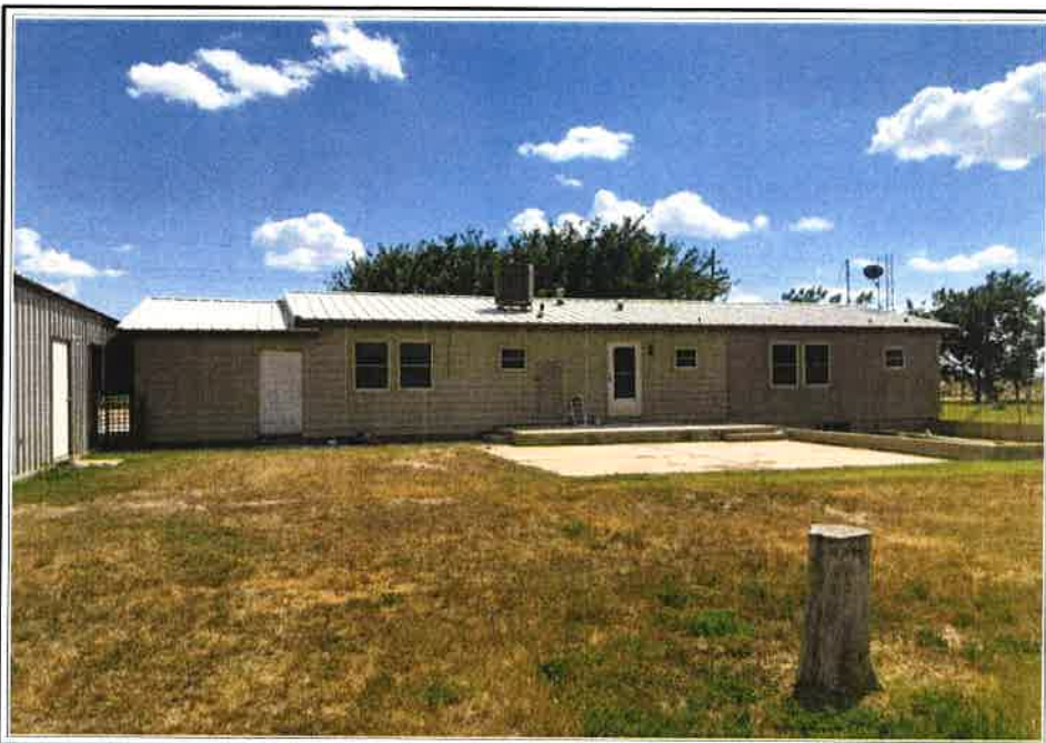
REAR OF SUBJECT PROPERTY
