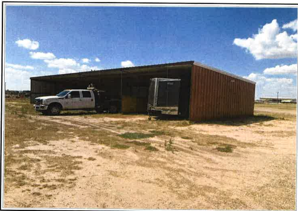
Additional Equipment Port
