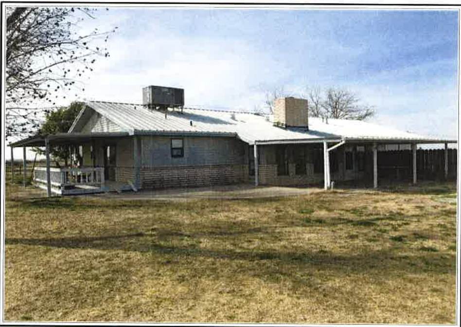
REAR OF SUBJECT PROPERTY
