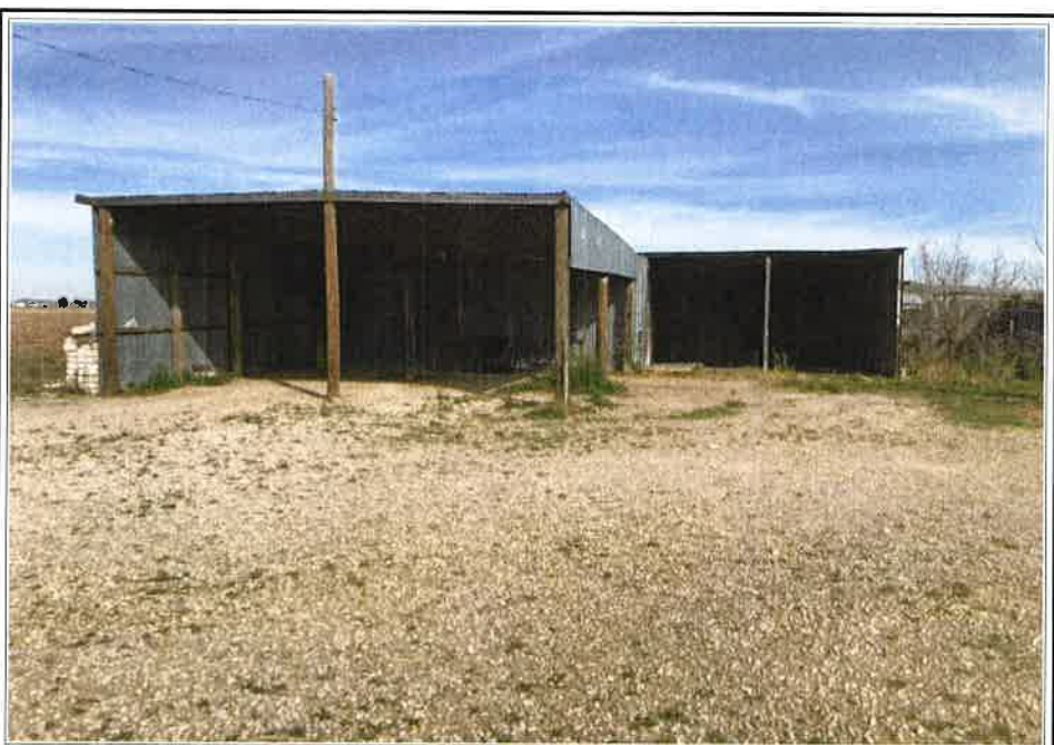
Open Barn, Storage barn
